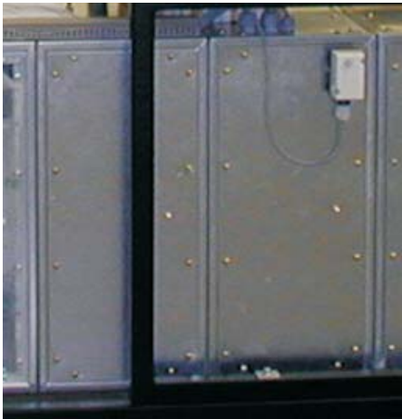
Fig. 2.9 From left, flow distributor and air heater with STL
