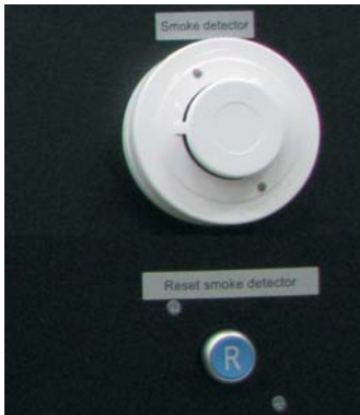
Fig. 2.22 Smoke detector with reset button
