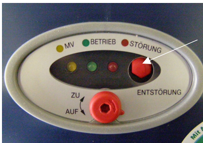
Fig. 2.5 Fault clearance button at burners housing
